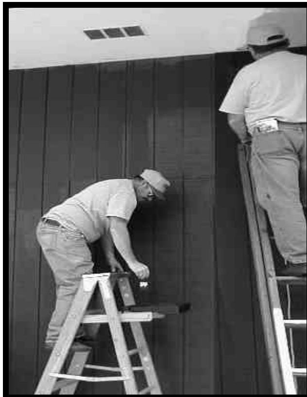
Cheerful Service. Willit's Dining Hall gets a fresh coat of paint by some Lodge Brothers.
