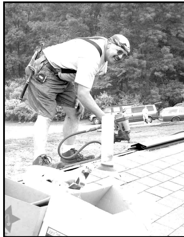
Another Day of Cheerful Service. Mike Ramich helps finish off a new roof on the former North Pool Bathhouses
